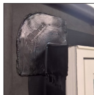
Fig 5: ME241 EPDM Corner applied to projecting window
